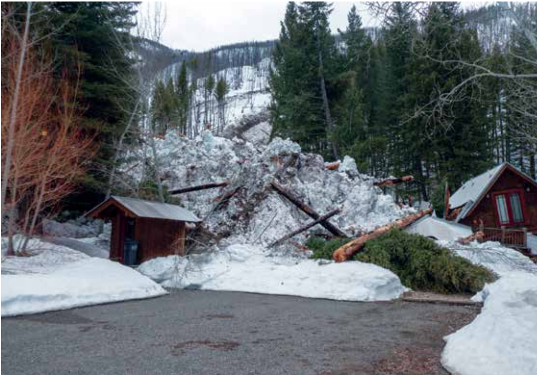
SAC: This is one of the two homes that were destroyed by wet slab avalanches west of Ketchum, Idaho. The main tongue of debris was an estimated 40' deep and packed with both live and burned timber well over 18" in diameter. Photo Sawtooth Avalanche Center
